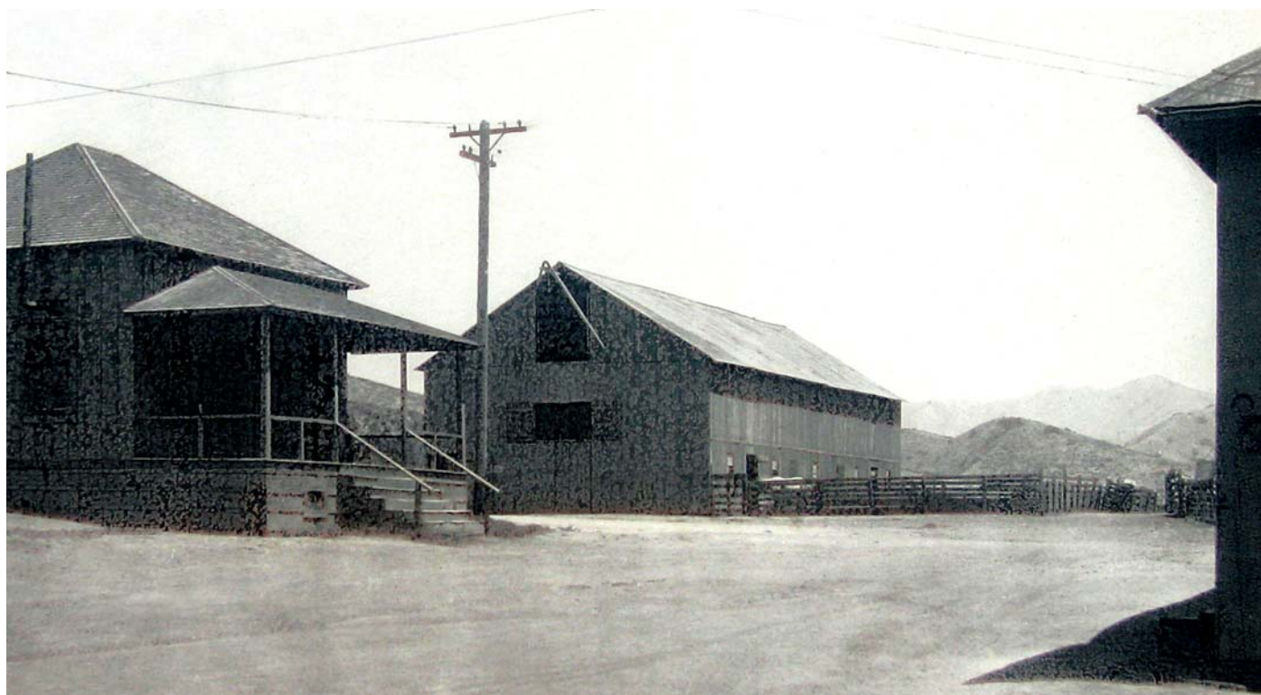
Middle Ranch as it appeared in the 1920s. This area is now the site of the Thompson Reservoir. Prior to building the reservoir, William Wrigley had the barn moved to the present site of the Conservancy's Facilities and Conservation Departments. The barn burned in 1990 resulting in the loss of several vehicles and tools.
